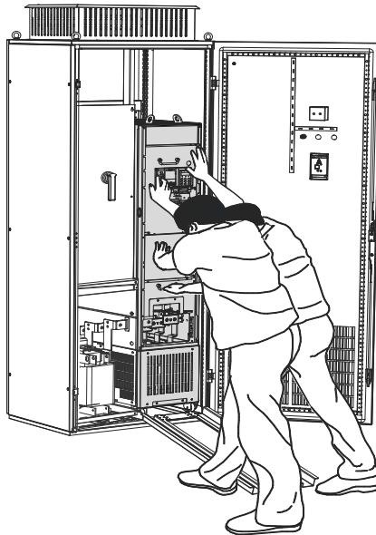
Figure 3-21 AC drive pushed into the cabinet
