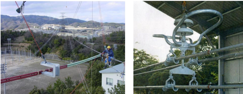
Fig. 2 Loading pipe between tower and cables (left) and clamp suspender (right).
